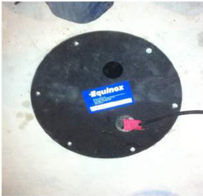
Identify sump pump area.
